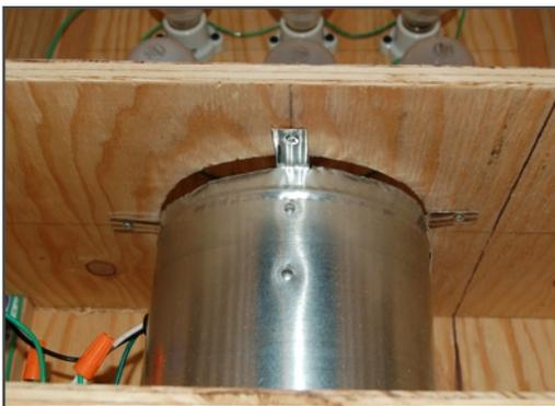
8. If you're using a duct-type fan, which I recommend, cut the necessary hole in the bulkhead (about 8 ½
