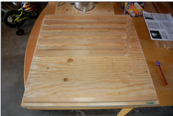
Figure 5. Cleats laid out on the inside surface
