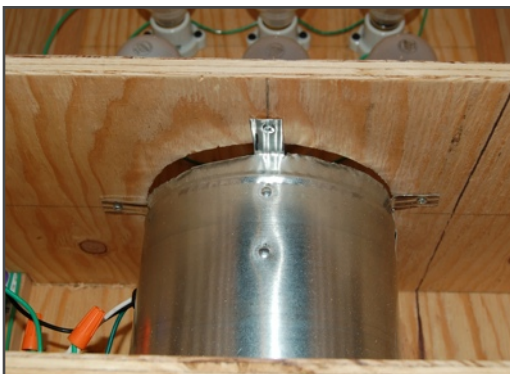
Figure 8. Fan mounted onto bulk-head via “tabs” made with tin-snips
